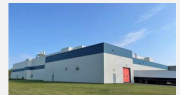
Production plant in Quebec, Canada
